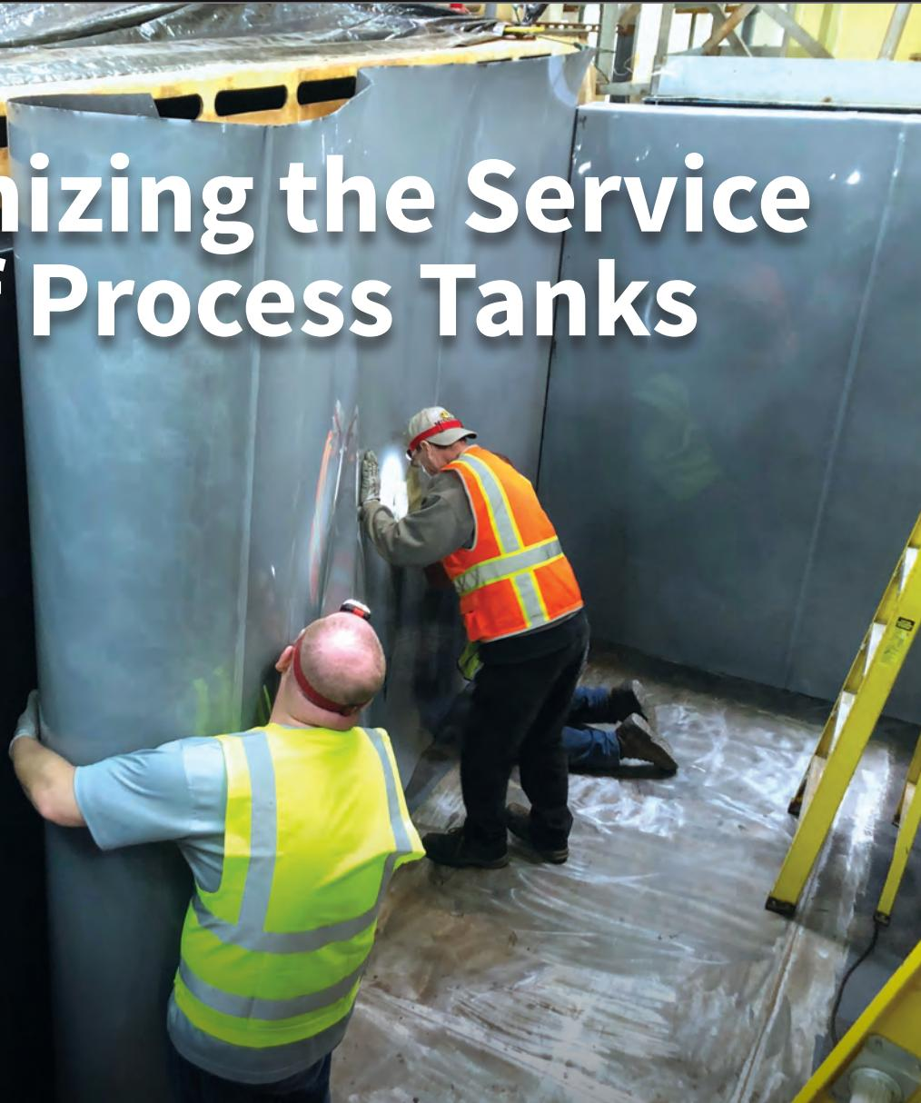
The most common materials used as process tanks include steel with a flexible polyvinyl chloride (PVC-P) lining or polypropylene (PP).
